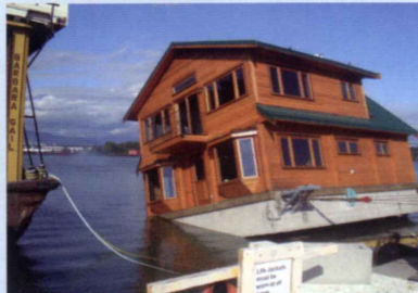
Maximum heel. A washer and dryer inside were well bolted down (the fridge was placed on its side for the occasion) and a piano which had been delivered just days before the launch was secured in the kitchen area with shrink wrap.
